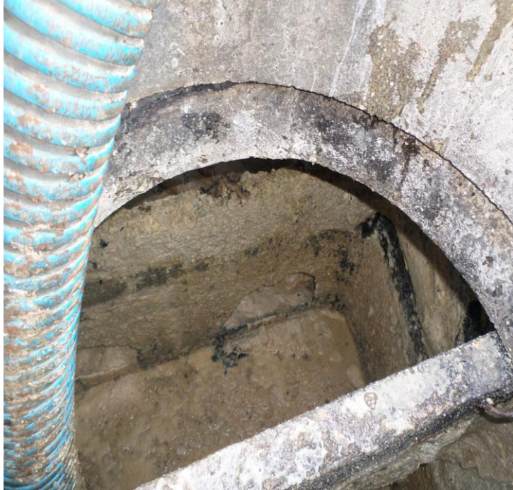
Damaged Baffle Popeye's
