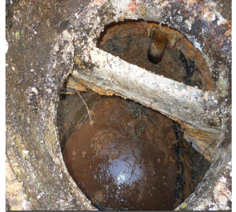
Damaged Baffle Mexican Villa
