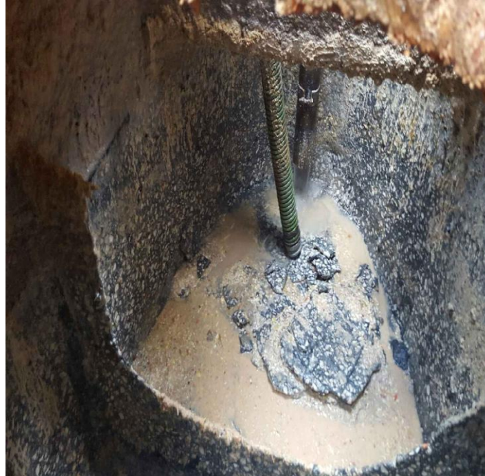
Collapsed Interceptor Garst
